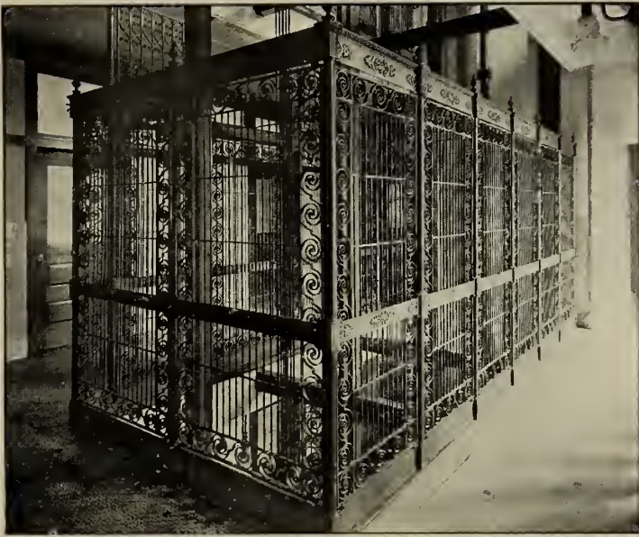
A.—ELEVATOR INCLOSURE, TEUTONIC BUILDING, CHICAGO. Wrought Iron, Bower-Barffed.
